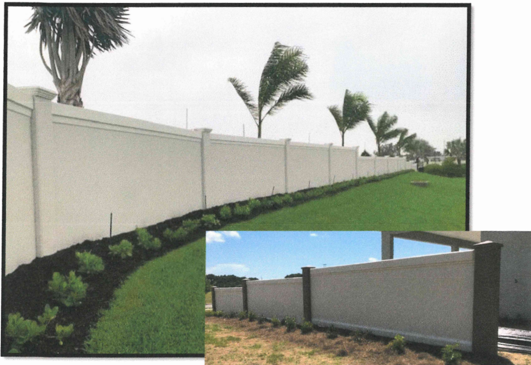
Example of proposed 6' tall precast concrete screen / buffer wall with 20' max column spacing. 2nd picture to show bottom banding / trim on the 6' panels.
